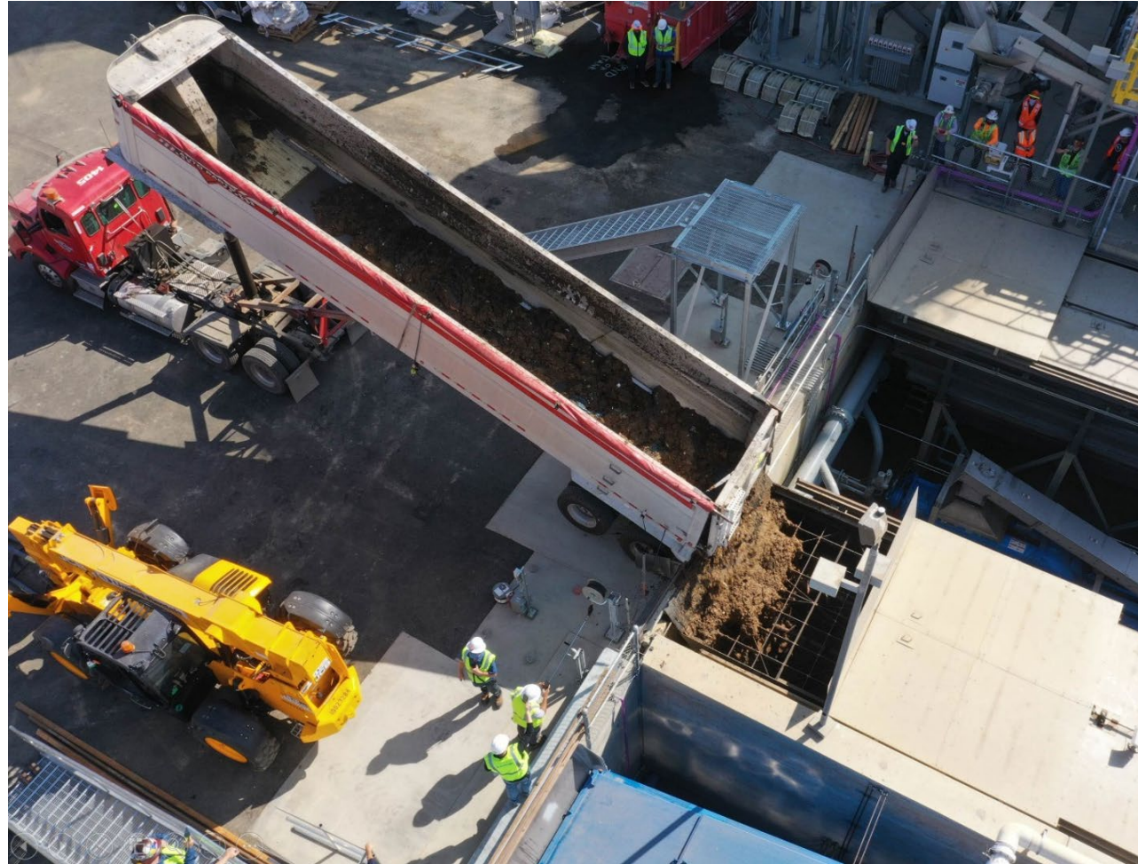
Organic fraction being delivered to Rialto Bioenergy Facility
