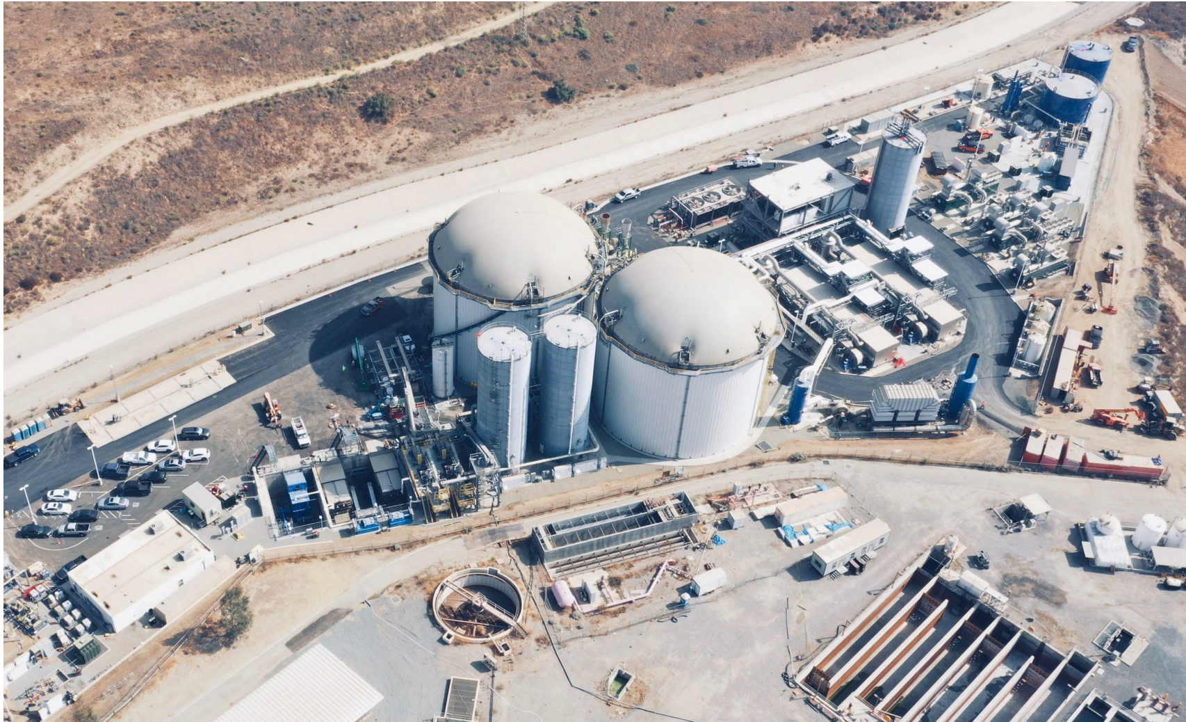
Rialto Bioenergy Facility
